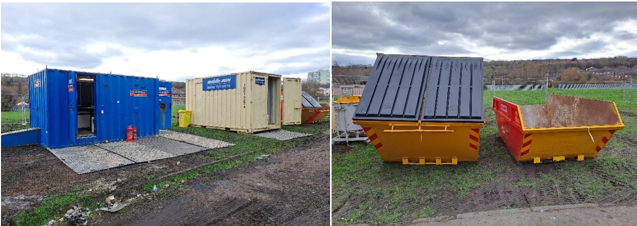
Fig. 5: Image taken of the site-setup completed in February 2023
