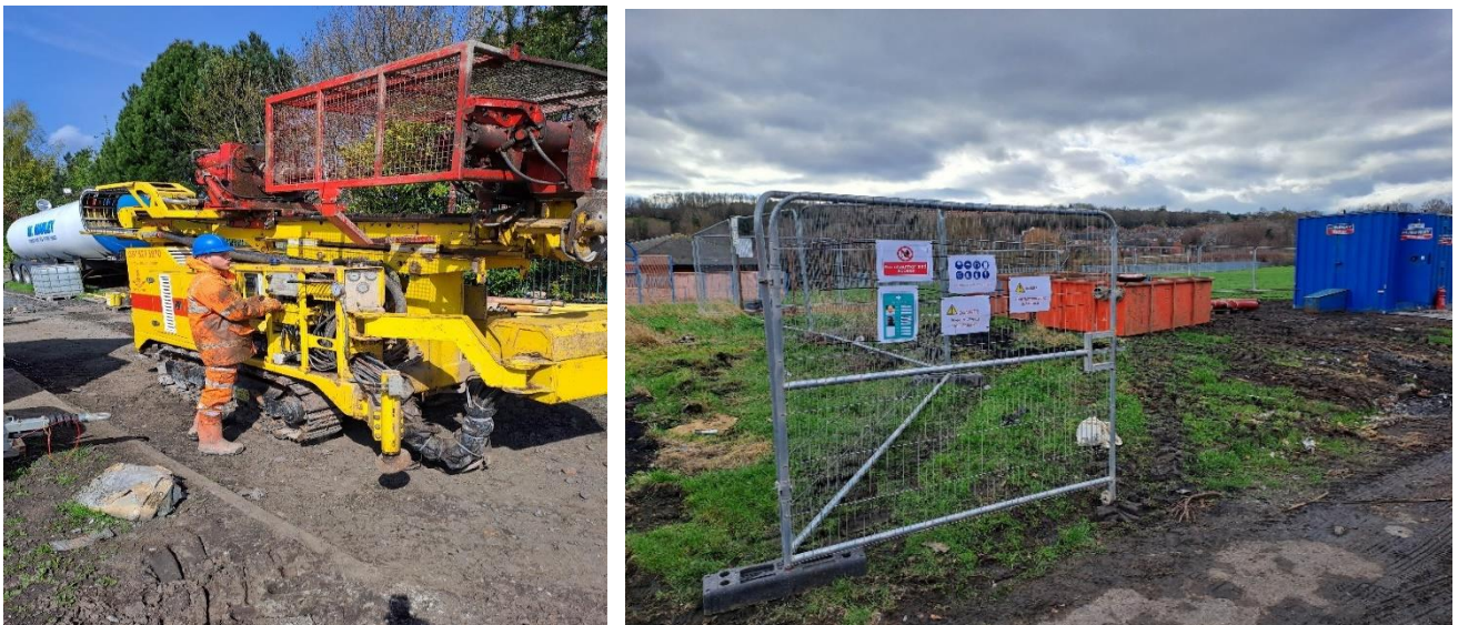
Fig. 6: Image taken of the site-setup completed in February 2023
