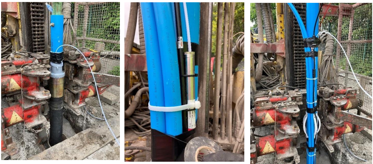
Fig. 10: Image acquired during the installation of the 4" casing and adjoining cables completed in June-2023
