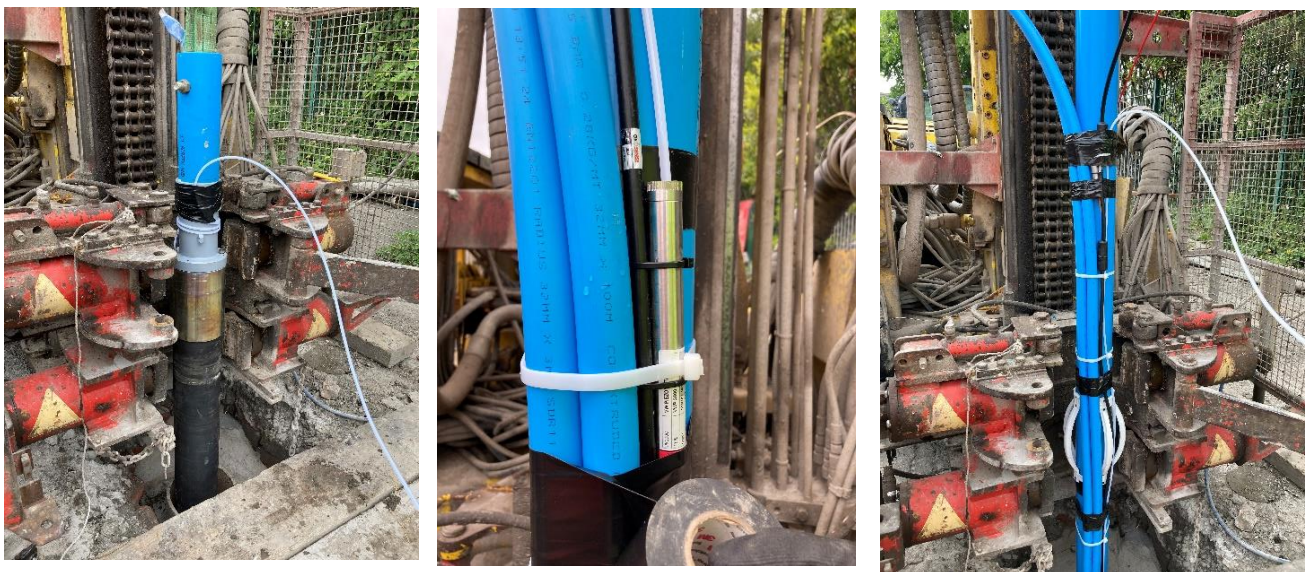
Fig. 10: Image acquired during the installation of the 4" casing and adjoining cables completed in June-2023
