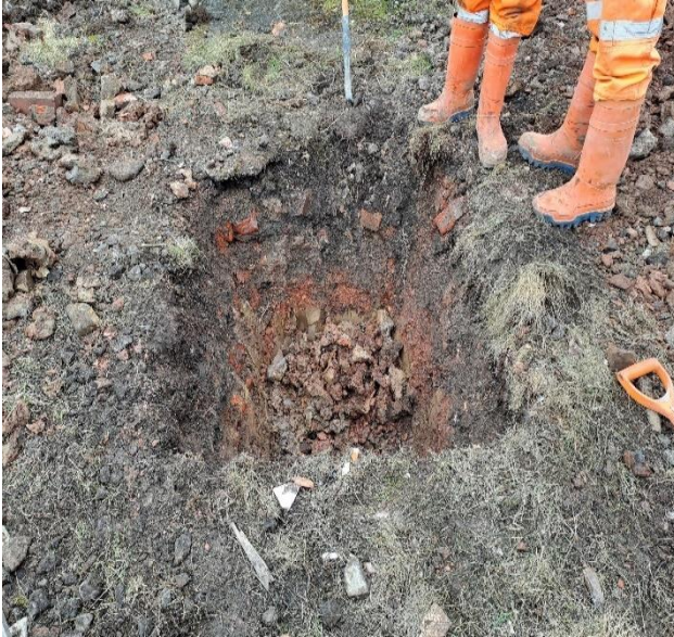
Fig. 7: Image taken of a trial pit being dug completed February 2023
